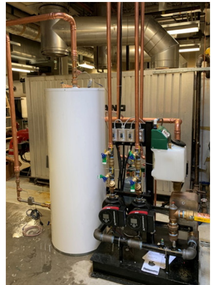
Figure 3: Left: Robur GAHP-A units installed on a rooftop. Right: Pump skid with a buffer tank and glycol feeder
