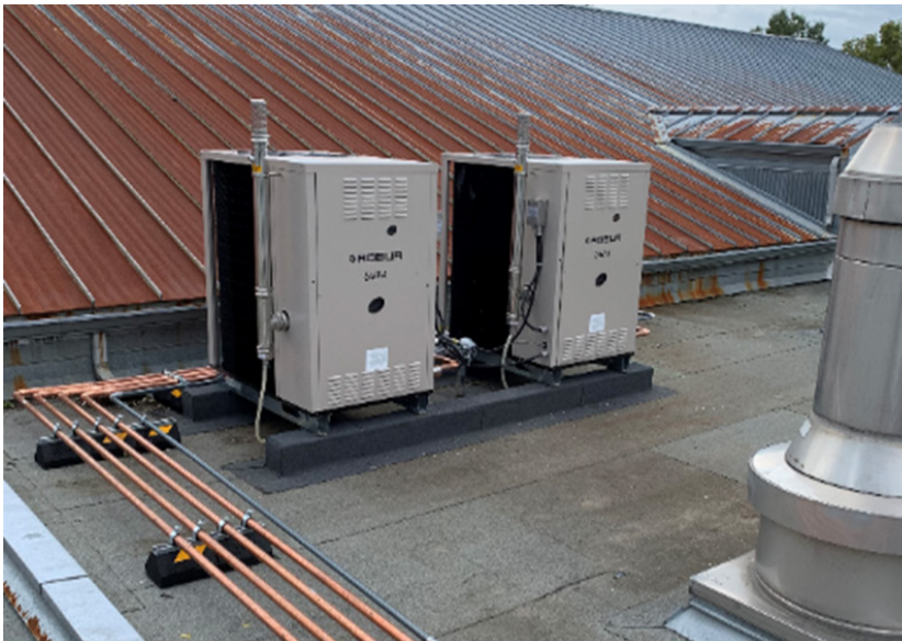
Figure 3: Left: Robur GAHP-A units installed on a rooftop. Right: Pump skid with a buffer tank and glycol feeder
